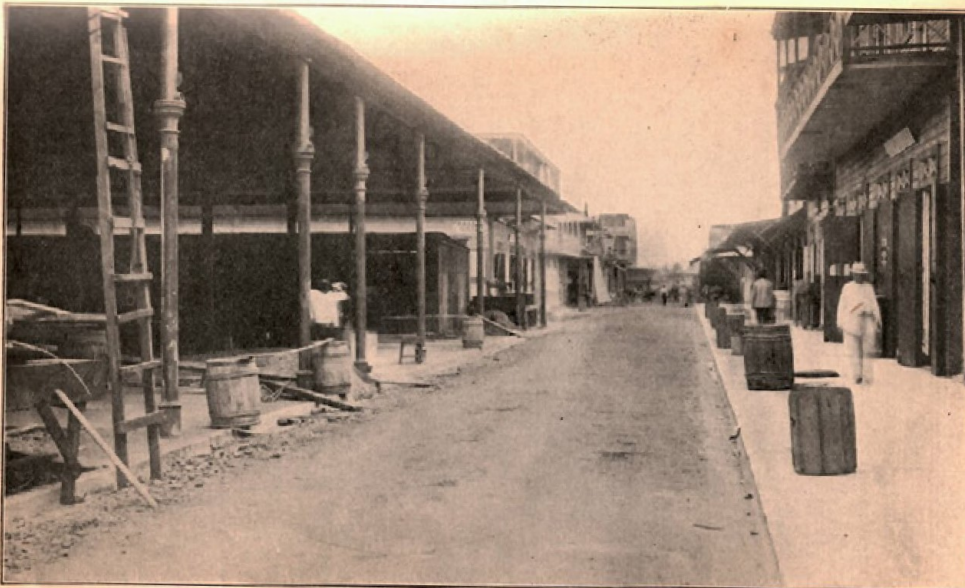
Fig. 34. View of Bottle Alley, Colon, June, 1907, Showing Proper Paving and Drainage Methods in the Canal Zone.
