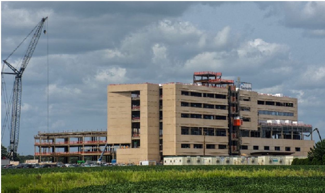
Figure 2. Construction of New Bayhealth Health Campus
